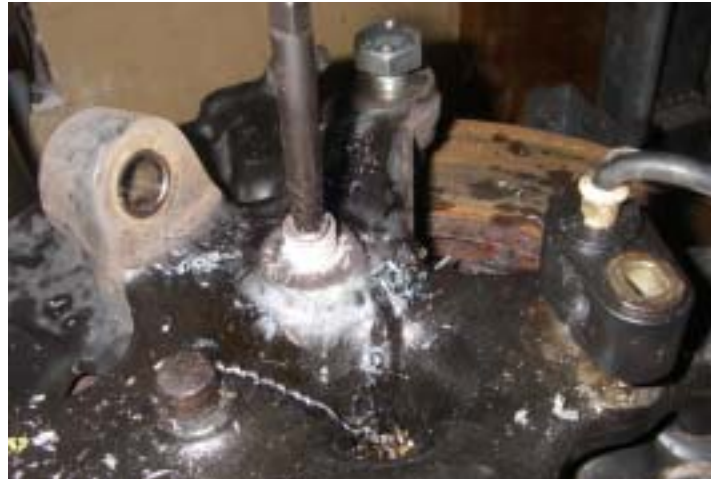
Photo #3 Removal of Broken Bolt
