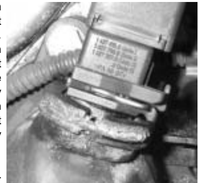
Photo #2 Leak Photo by Vic Lucariello, Sr.
