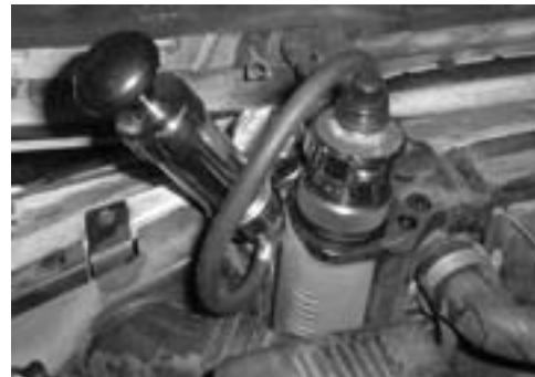
Photo #3 Better View of Pressure Test Vic Lucariello, Sr.
